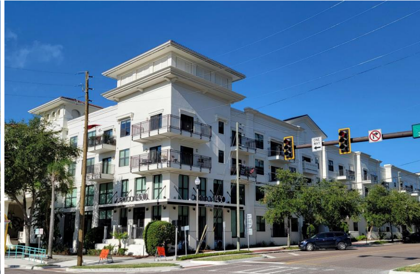
The Beacon at 340 | 75 units per acre
